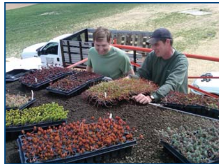
Joppatowne High School students and the HCPS facilities crew install a living green roof on top of the school's new concession stand.
