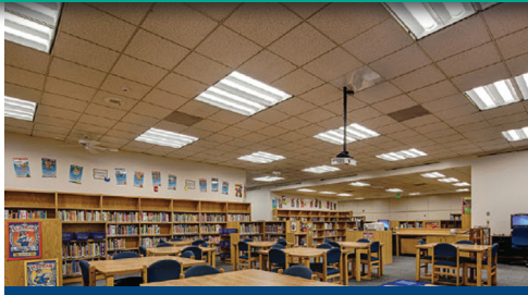
Sensors in Prospect Mill Elementary School's library enable lighting by zones for use by small groups.
